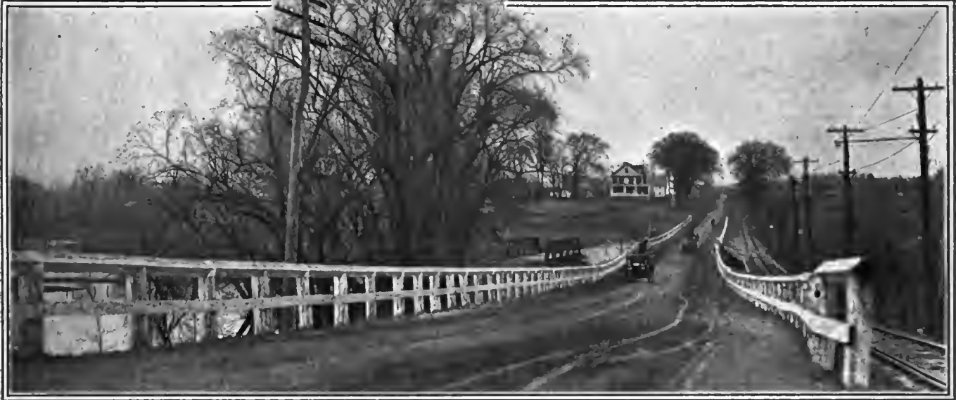
This illustration shows how the State of Connecticut got rid of a dangerous turn in the highway by changing the course so that the road is straight. The old iron bridge at the left of the white fence was formerly used
